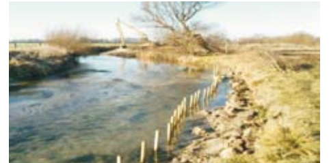
Left: Large woody debris (LWD) was inserted into the new bank line to enhance flow diversity. The logs were securely pinned to the river bed. Right: Removal of the stone weir was undertaken and the stones and silt have been placed behind the nearby bank revetment. The new line of the bank was marked by pressing in posts where the willow spiling will be woven.
