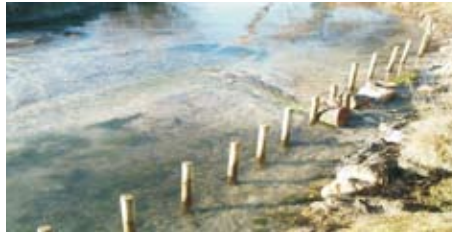
Left: Large woody debris (LWD) was inserted into the new bank line to enhance flow diversity. The logs were securely pinned to the river bed. Right: Removal of the stone weir was undertaken and the stones and silt have been placed behind the nearby bank revetment. The new line of the bank was marked by pressing in posts where the willow spiling will be woven.
