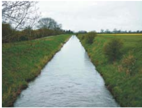
Upstream section at Brompton
