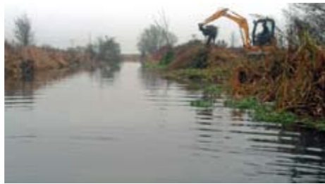
Backfilling of new 'D' shaped submerged berm
