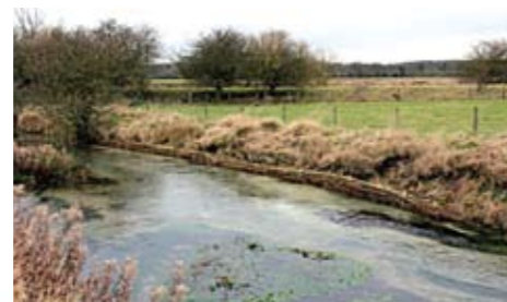
Willow spiling used to protect the toe of the eroded bank. The small island has been retained to maintain the narrow channel and both banks have been protected from increased erosion
