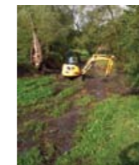
Stream restoration works autumn 2014
