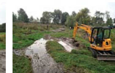
Creating new sinuous low flow central channel
