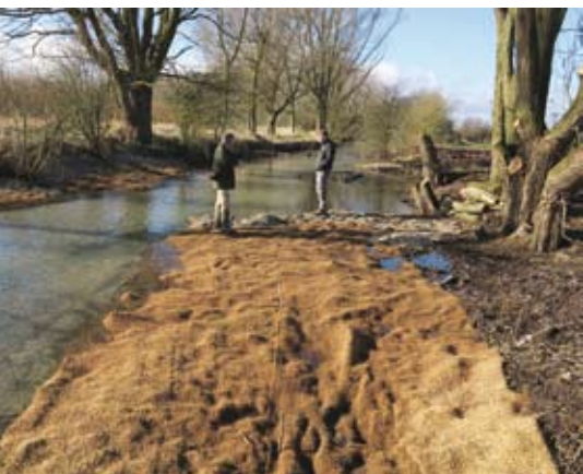
Left: Coir matting protecting the new bank
