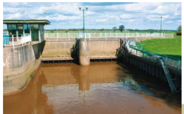
Barmby Barrage – where the Derwent joins the River Ouse. There are migration issues with this structure
